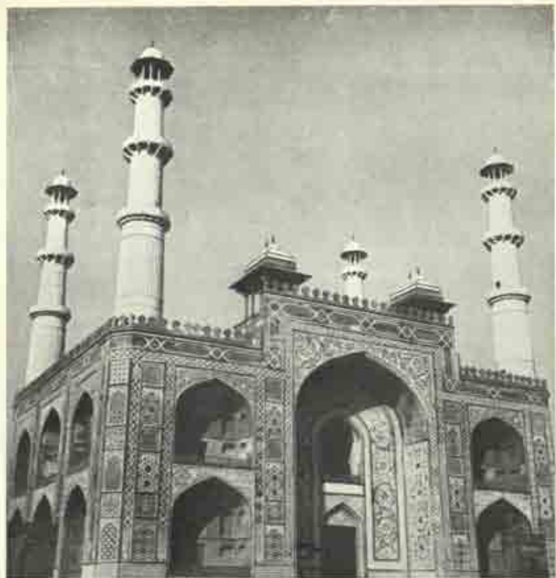
10. Facade, Southern gateway, Akbar's tomb, Sikandara.
